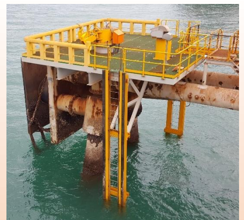
Platform refurbishment complete with new hook assemblies and access ladder installed
