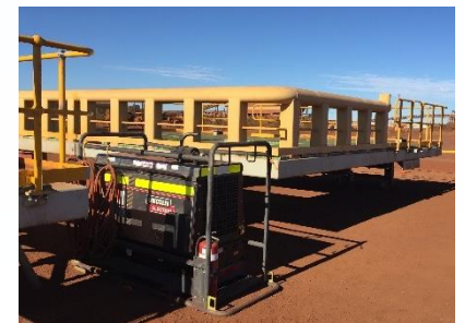
Platform pre-assembled with all non destructive testing completed
