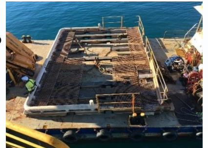
Redundant Dolphin platform loaded onto Multi-Cat via crawler crane
